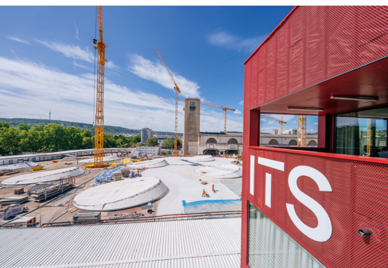
You couldn't get any closer to the action: the InfoTurmStuttgart is located right in the heart of the construction site.
